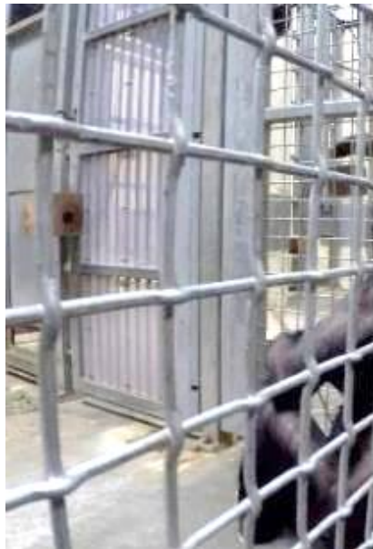
Figure: 13: Steel crimped mesh welded in a steel frame
