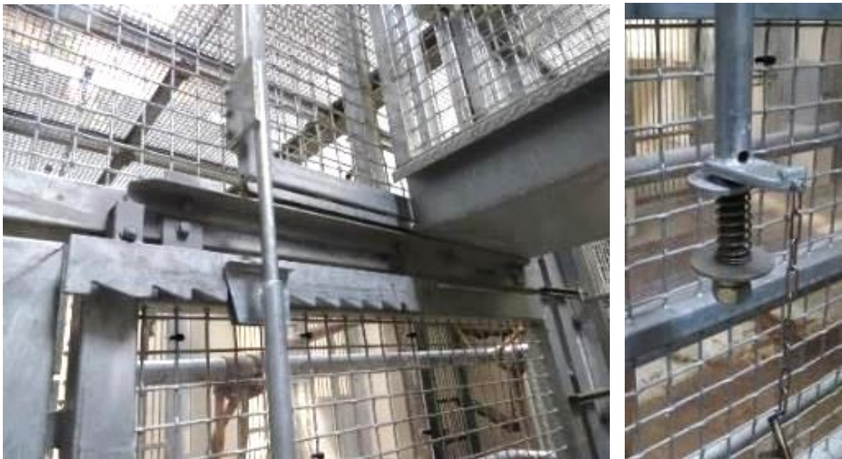
Figures 21 & 22. Sliding door that moves along a strip with teeth, fixed to the fence construction.
