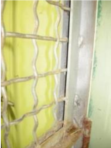
Figure: 14. Wave mesh welded between steel profiles (Photo: G. Fernández Hoyo)
