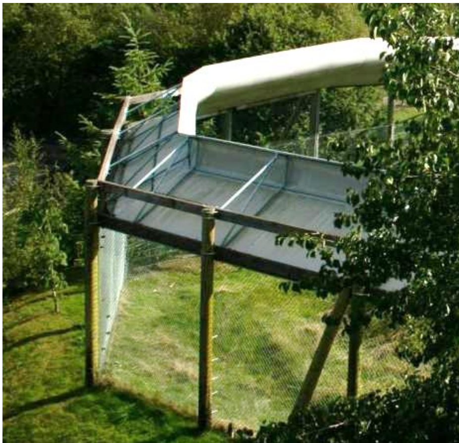
Figure: 17: Special overhanging structure as containment on a chain-link mesh fence at Monkey World (Wareham). Note the hotwires to protect the chain-link mesh.
