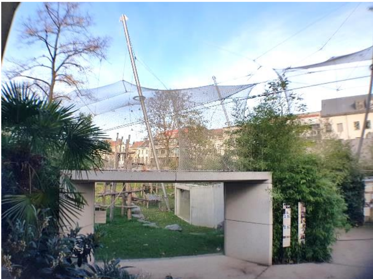
Figure:18. Stainless steel net was used for the chimpanzee enclosure at Antwerp Zoo
