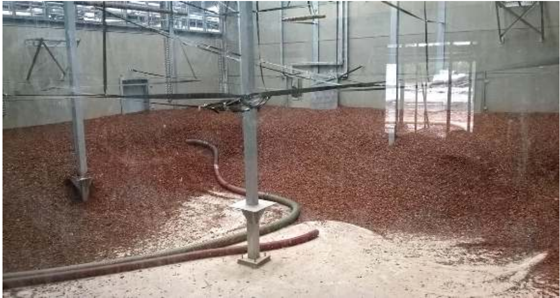
Figure: 25. Installing the bio-floor at Twycross Zoo (Photo Twycross Zoo)
