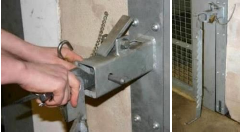
Figures 19 & 20. Sliding door with teeth on the handle as applied for orangutans at Chester Zoo.
